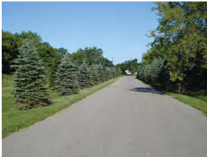
Wolcott Mill Estates Entrance Roadway - reduced roadway width with open ditching
