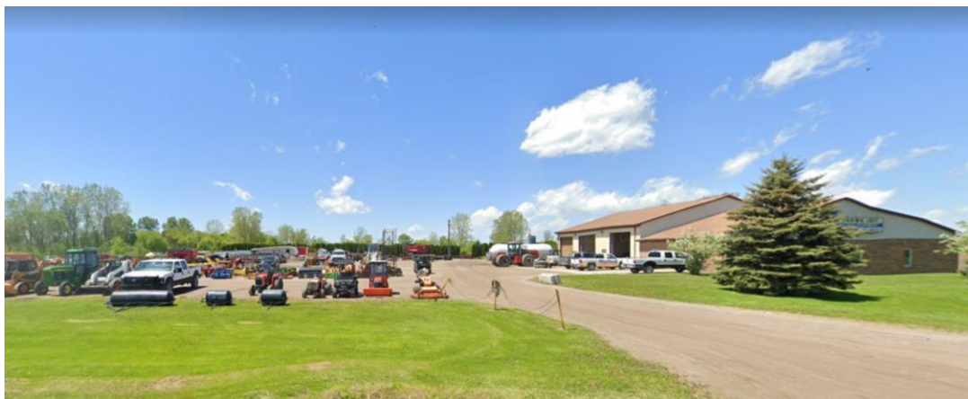
View of Property Looking West from North Avenue
